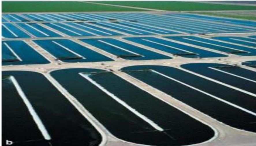
Figure 11: Culture de Spiruline en raceway, Californie (Andersen, 2005).
