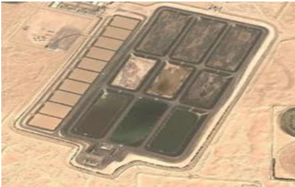
Figure 7 station de lagunage aéré de HASSANI ABDEL KARIM.
