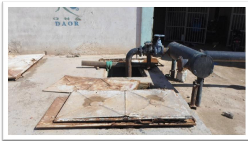
Figure 7: photo station de relevage
